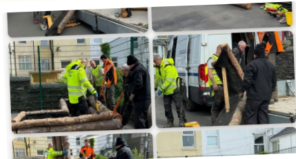
Pond going in, with Douglas City Council
